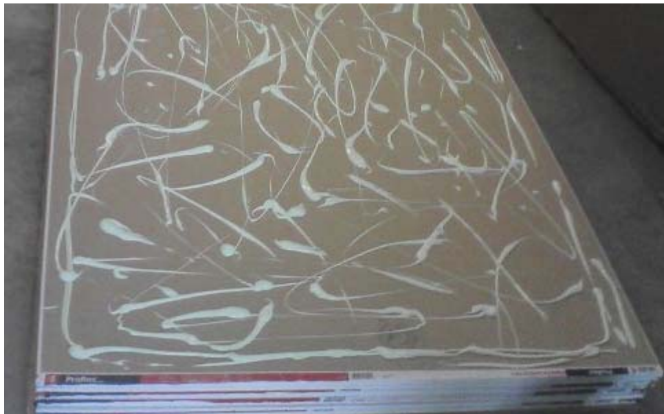
Figure 1: Typical glue application pattern (photo supplied by Client)
