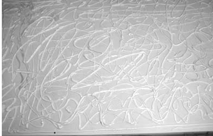
Figure 2: Typical glue application pattern (photo supplied by Client)
