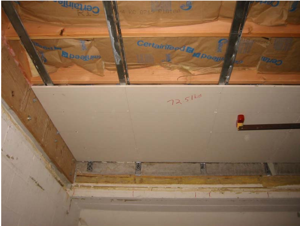
Figure 2: Joists, insulation, resilient channel and partially installed ceiling
