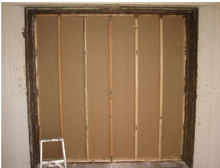
Figure 2: Green Glue® Noiseproofing Clip RC Layout Photo
