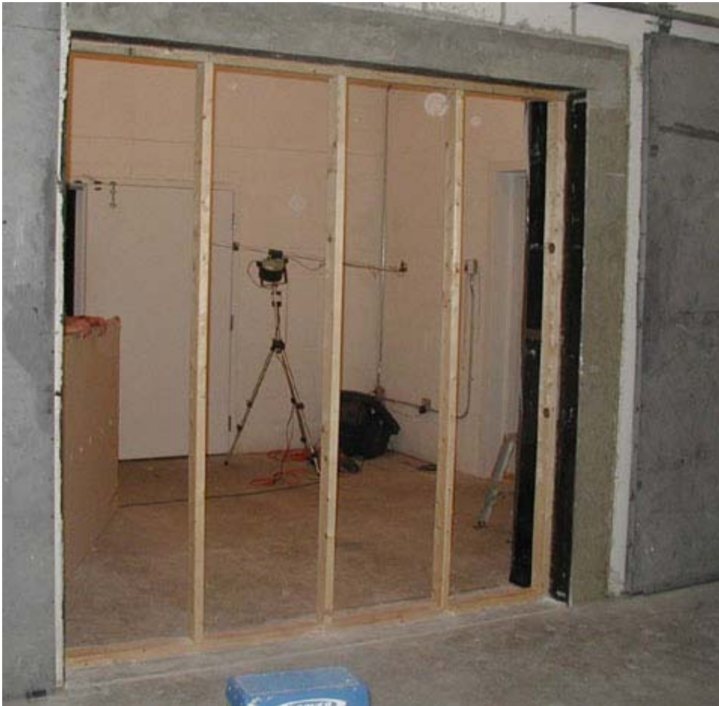
Figure 2: Wood-stud Specimen Frame in Opening
